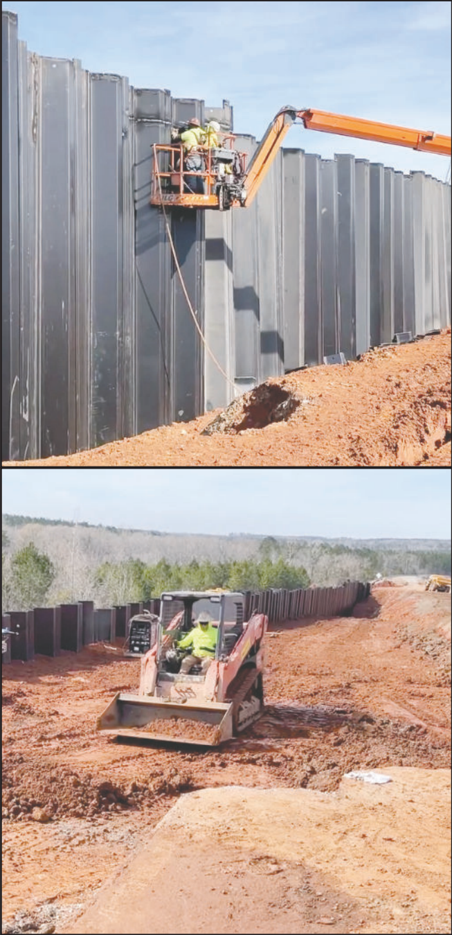
Courtesy of Georgia Department of Transportation
