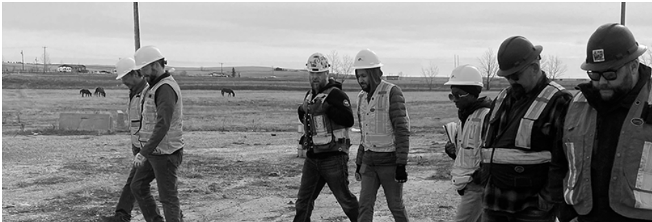
Cluny Demolition Project: Pre-Kick-off Meeting Phase 2 initiated following take-down of former Crowfoot residential school building, site of the former school grounds including Parrish Hall and school yard. The next phase of the project is topsoil remediation and restoration.
