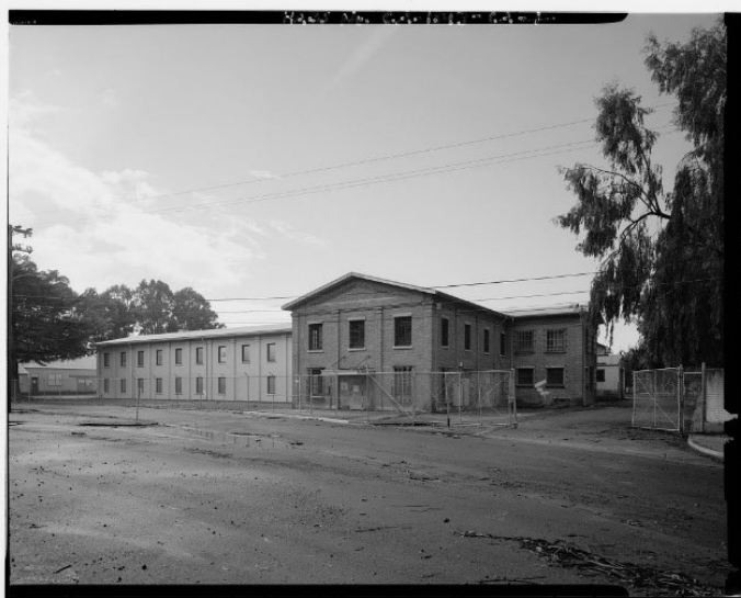
Southwest view of the Naval Retraining Command, otherwise known as building 84, or "Old 84." Library of Congress Images.
