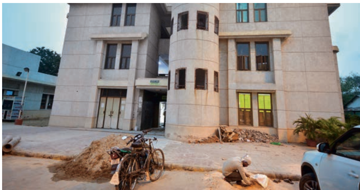
CONSTRUCTION WORK in full swing for a COVID vaccine storage unit at the Rajiv Gandhi Super Speciality Hospital in New Delhi, on December 20, 2020.
