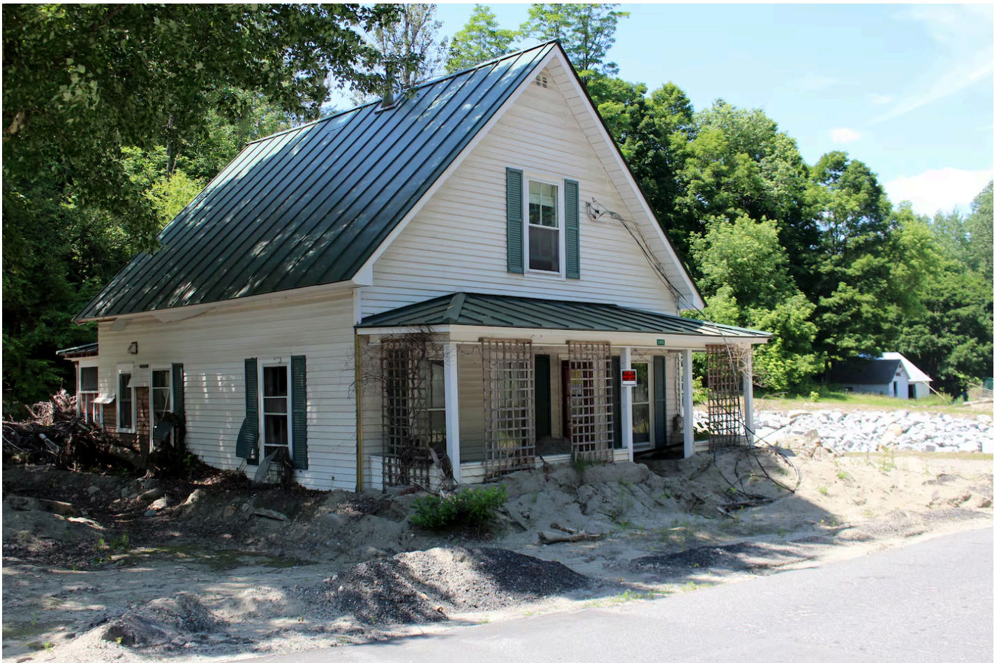
A house in Plainfield, Vt., remained covered in dirt and silt earlier this month as the owners awaited word on government buyout programs. PAUL HEINTZ FOR THE BOSTON GLOBE
