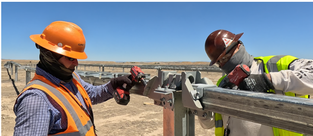
Figure 1: Technicians utilizing Milwaukee's CTIW on the Nevados tracker in the field
