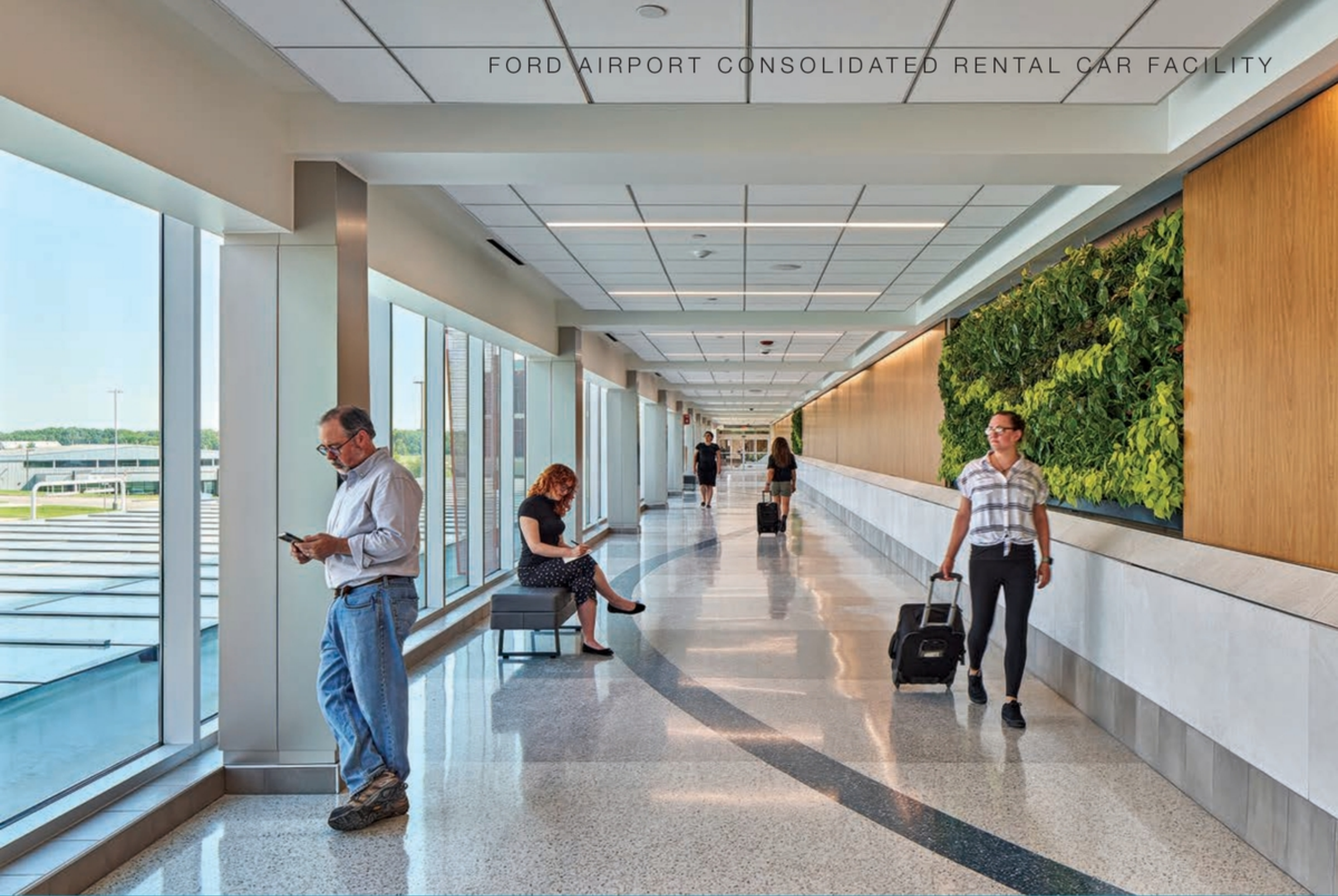
An enclosed skybridge stretches between the ConRAC and terminal, creating a weather-protected passenger route while crossing an active airport roadway. Portions of the skybridge ceiling and exterior wall were prefabricated to shorten field installation time and reduce overhead congestion. Photo credit: Maconochie Photography
