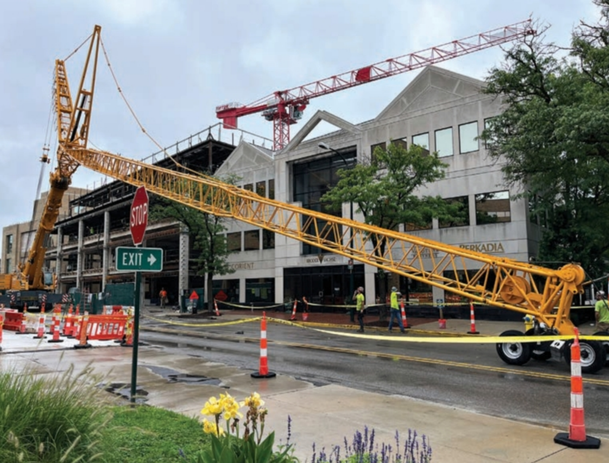
Construction of 370 Brown unfolded within the tight confines of downtown Birmingham, requiring careful coordination of cranes, equipment, deliveries, and street access while work continued alongside neighboring buildings and businesses
